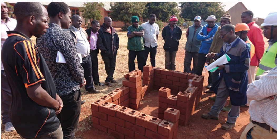
Lyra's main contractor, Pato Ninje explaining the production and benefits of ISSBs
